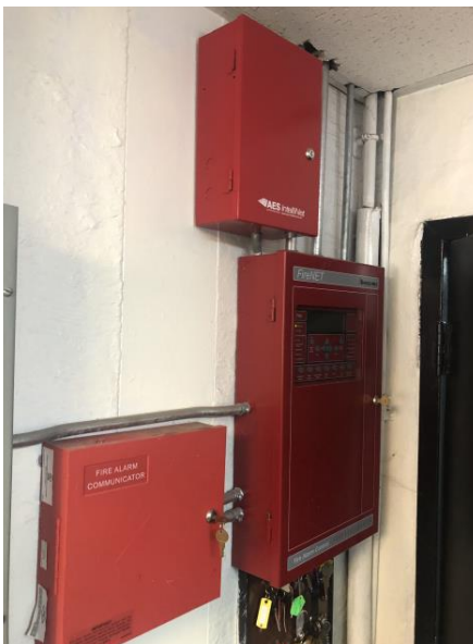
Existing Fire Alarm Control Panels
