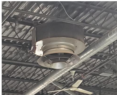
Existing Vertical Unit Heaters
