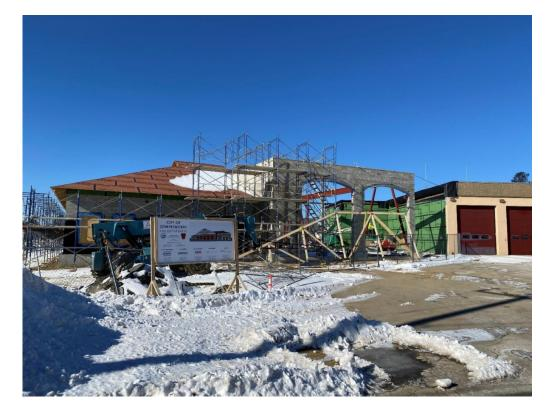
Phase I construction of Somersworth's New Fire Station continues as the roof is nearing completion on the logistics wing and masonry work for the first two apparatus bays is progressing.
