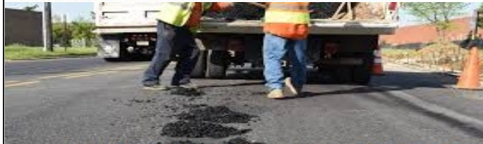
Currently Applying Temporary Cold Patch from rear of dump truck
