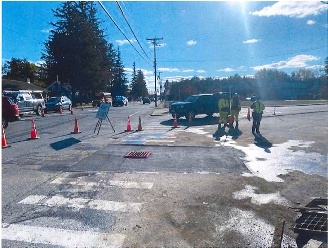
Blackwater Water at High Street stormwater structure replacement
