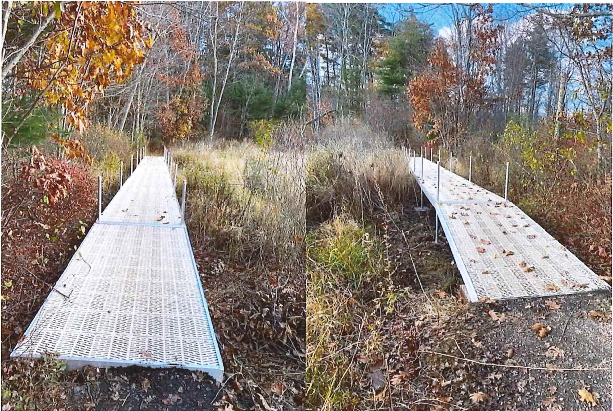
New trail bridges replaced at Willand Pond.
